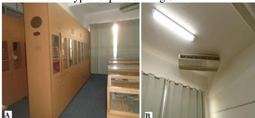
Fig.3. Showing storage cupboards and air-conditioning devices; A-showed that the storage cupboards do not contain temperature and relative humidity measuring devices; B- showed the air-conditioning devices have no filters.
